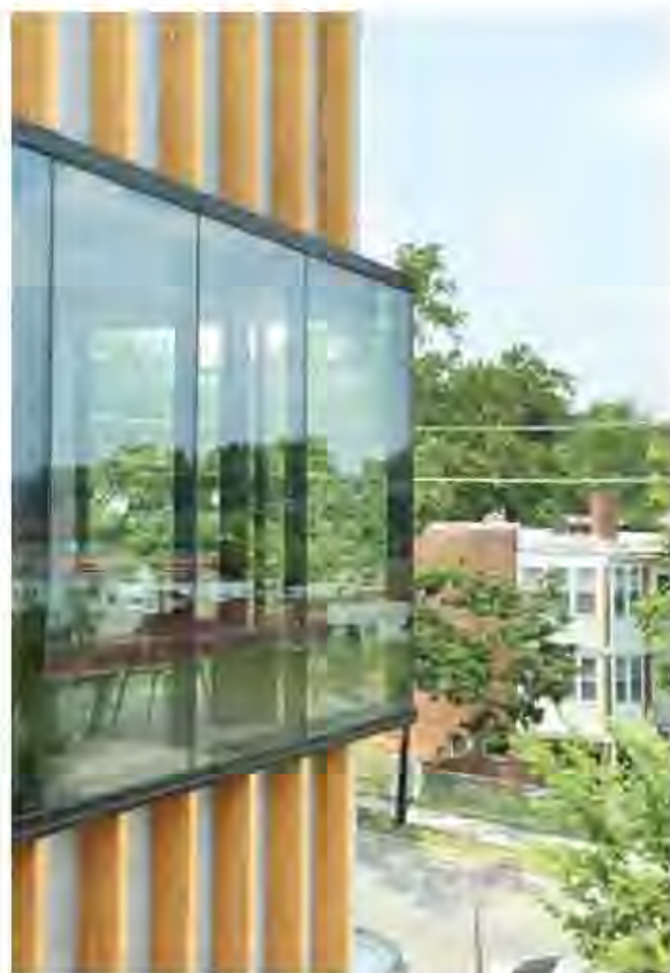
In the William O. Lockridge/ Bellevue Library the facades have been created with a combination of concrete sections, large glass surfaces and Parallam-type wooden slats
